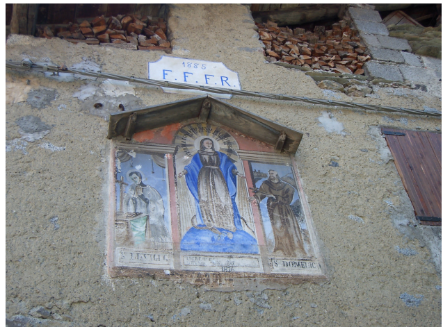
in via Mazzini - Garda
